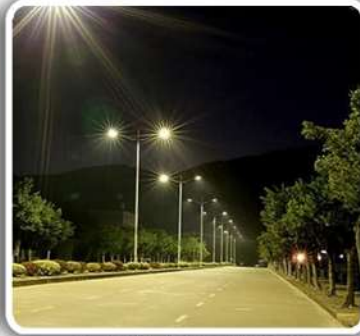
STREET LIGHTS & 24 HOURS ELECTRICITY
