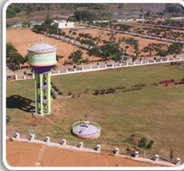
OVER HEAD WATER TANK
